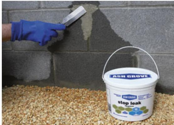
**Ash Grove® Stop Leak is an extremely rapid-setting cement repair material designed to stop the flow of water leaking through cracks and holes in concrete and masonry.**
