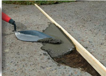
**Ash Grove® Sand Mix is a uniformly blended mixture of Portland cement, sand and other approved ingredients designed for general concrete repairs.**
