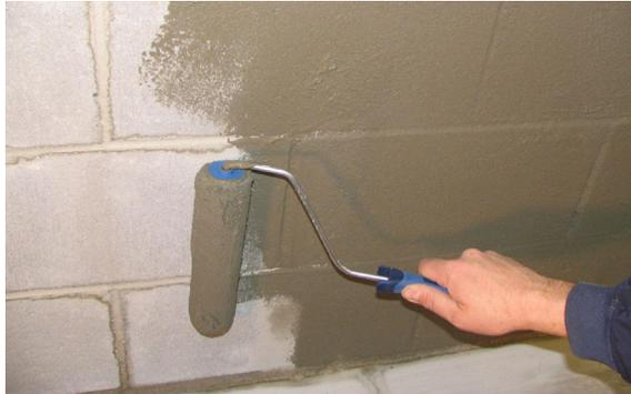
**Ash Grove Pro® Wall – Tite Unsanded is a polymer modified, waterproof cement coating for above and below ground concrete and masonry surfaces. Ash Grove Pro Wall-Tite Unsanded is recommended for waterproofing, basements, cisterns, foundations, reservoirs, silos, and grain elevators.**
